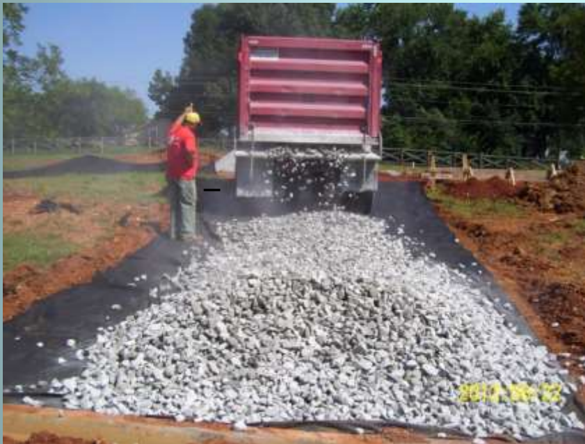
Construction Exit Pad
